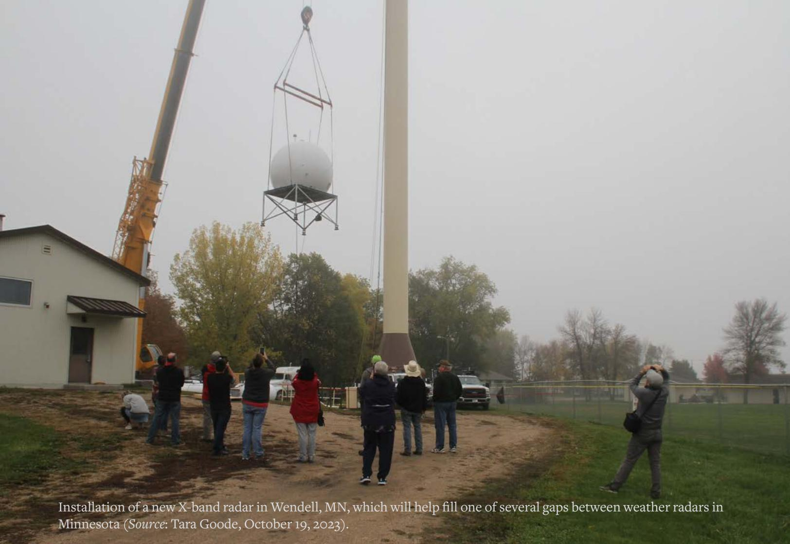
Installation of a new X-band radar in Wendell, MN, which will help fill one of several gaps between weather radars in Minnesota (Source: Tara Goode, October 19, 2023).
