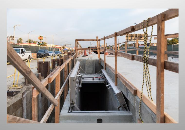
A new 8.5-mile, \$2.058 billion rail line is being constructed in Los Angeles, California. The project includes several underground stations, where access doors have been installed to meet NFPA codes for emergency egress (*Source:* Photos by Dan Arnold, February 2018).
